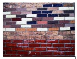
Depending on their material and the firing method used, bricks can be a variety of different colors.
